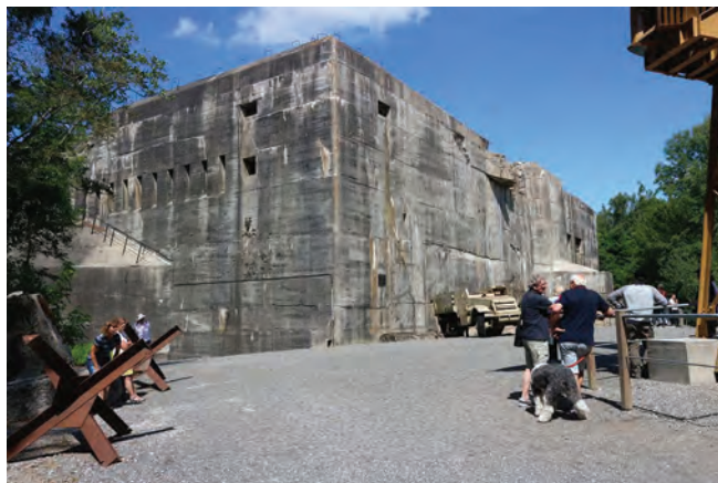
The western and southern faces of the blockhouse. Photo Bob Clary
